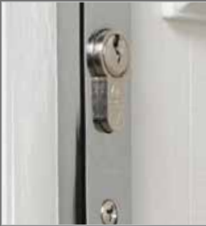
Ultra high-security cylinder lock
